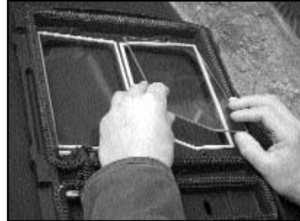
Fig 9b fitting new glass
