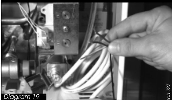
The mains electrical cable is supplied with the boiler. It is coiled and tucked inside the boiler
