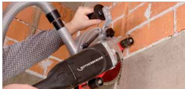
Effort-saving operation with the downward pulling cut
