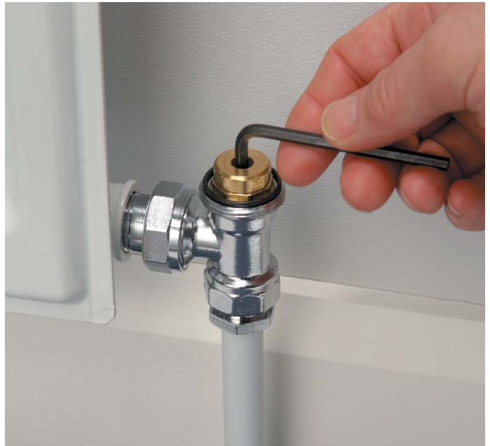
Tamper resistant lockshield adjustment by allen key
