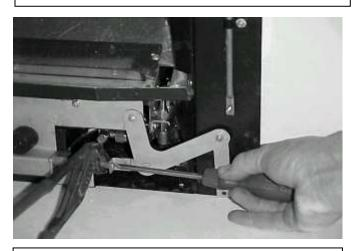
Check for gas soundness. Reconnect the bell crank mechanism as above ensuring that the gas control spindle is gripped only over the protective copper sleeve and no other part of the spindle as, ensure NO side strain is applied to the spindle.
