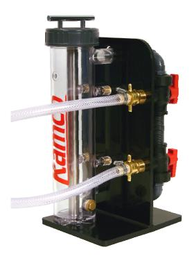
The CombiMag filter increases power flushing efficiency by removing circulating black iron oxide contamination from the system water. The filter is simply installed in line between the heating system and the power flushing pump.
