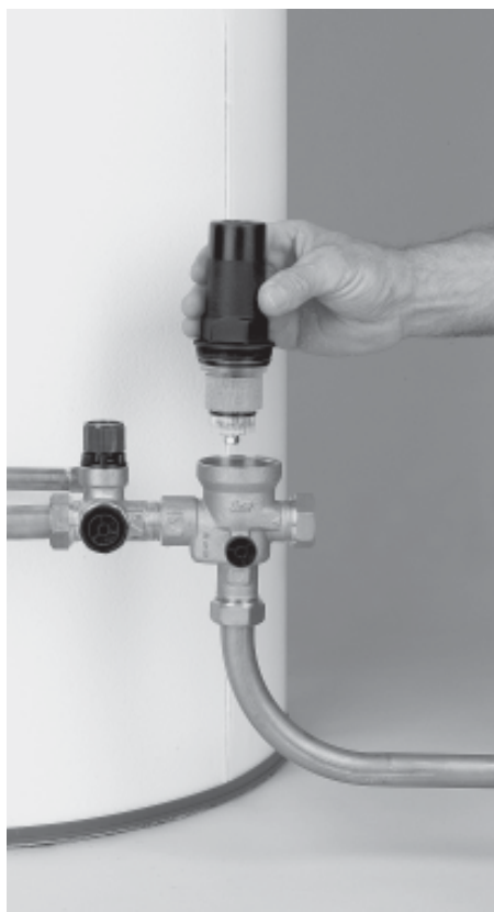
Fig. 4 Remove the filter from the inlet control set.
