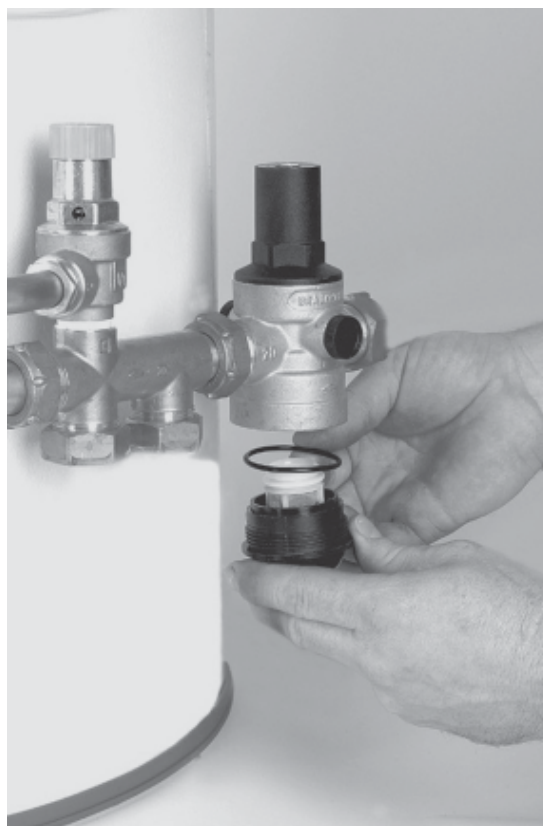
Fig. 5 Clean the filter and refit.
