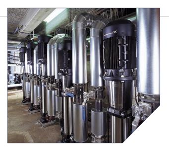
and do not require any additional tank to provide supplementary pressure. In boiler feed applications, where many big tanks are gathered, a compact system is an advantage.
