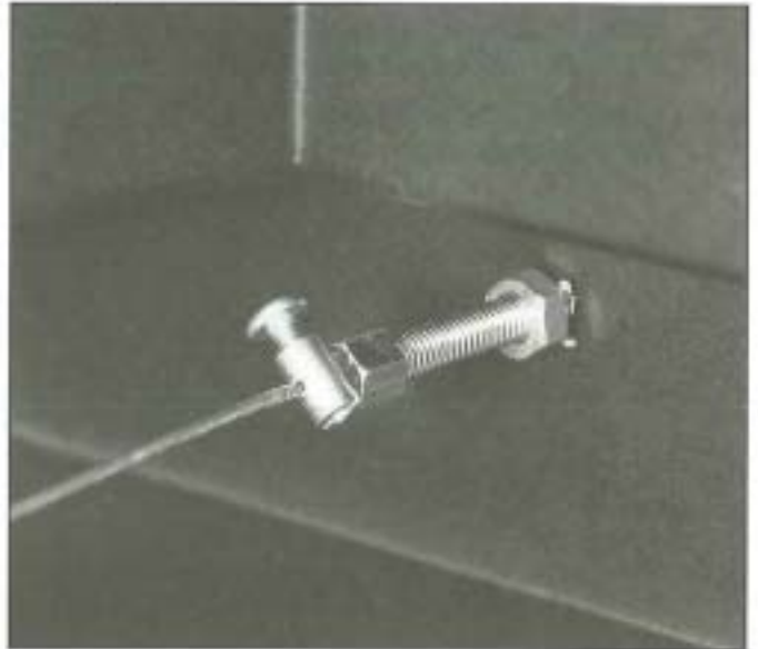
FIG 8 Tensioning bolt extended, firmly securing the appliance into the opening with the sealing strip compressed between the fire-box frame and the fireplace.
