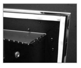
SCREW FIXING. For fixing by screw, mark and drill the fireframe or base, and the relevant points in the opening or on the wall. Rawlplugs will again be required. Pre-punched holes are not provided for this purpose to allow you to choose the optimum positions.
