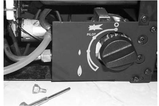
2) On the valve above the control knob. Remove the data plate by unscrewing the two retaining screws. There are two pressure test points above the control knob. Remove the screw from the LEFT hand nipple, marked 'OUT' and attach a U gauge.
