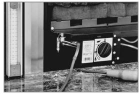
If the pressure is too low, then check the meter governor pressure with the appliance running. If this is incorrect it will need to be reset by the gas supplier.
