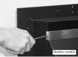
Protect the decorative hearth whilst pushing the convector box in and out of the opening. Part of the packaging is an ideal hearth saver pad.
