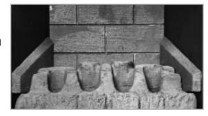
Place the front row of six coals on to the matrix, with the two coals second front each end turned on their sides. Ensure the coals are firmly against the side cheeks as shown in the photograph. If necessary, pull the coals forward slightly to ensure their rear edges do not overhang the flame ports. Corners or rough edges MUST NOT be allowed to enter the flame ports.
