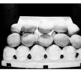
4. Now take another two pebbles and place behind the second row of coals, next to each other in the centre of the fuel bed. The pebbles may be orientated as desired to achieve a realistic effect. Keep the spacing between the pebbles even and uniform.
