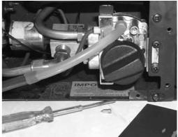
If the pressure is too low, then check the meter governor pressure with the appliance running. If this is incorrect it will need to be reset by the gas supplier. If the setting pressure is too low, but the meter pressure is acceptable, then a problem in the supply pipework is to be suspected. This will be dirt and debris, kinked or inadequate size pipes, restriction in a fitting or solder flashing across a joint.
