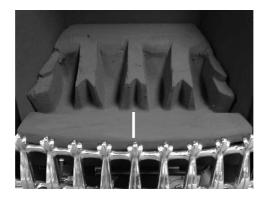
Fit five of the large sized coals onto the front ceramic rail, ensuring that they are evenly spaced. Use the recess's in the front ceramic rail as a guide for placement. (See fig. 12 below)
