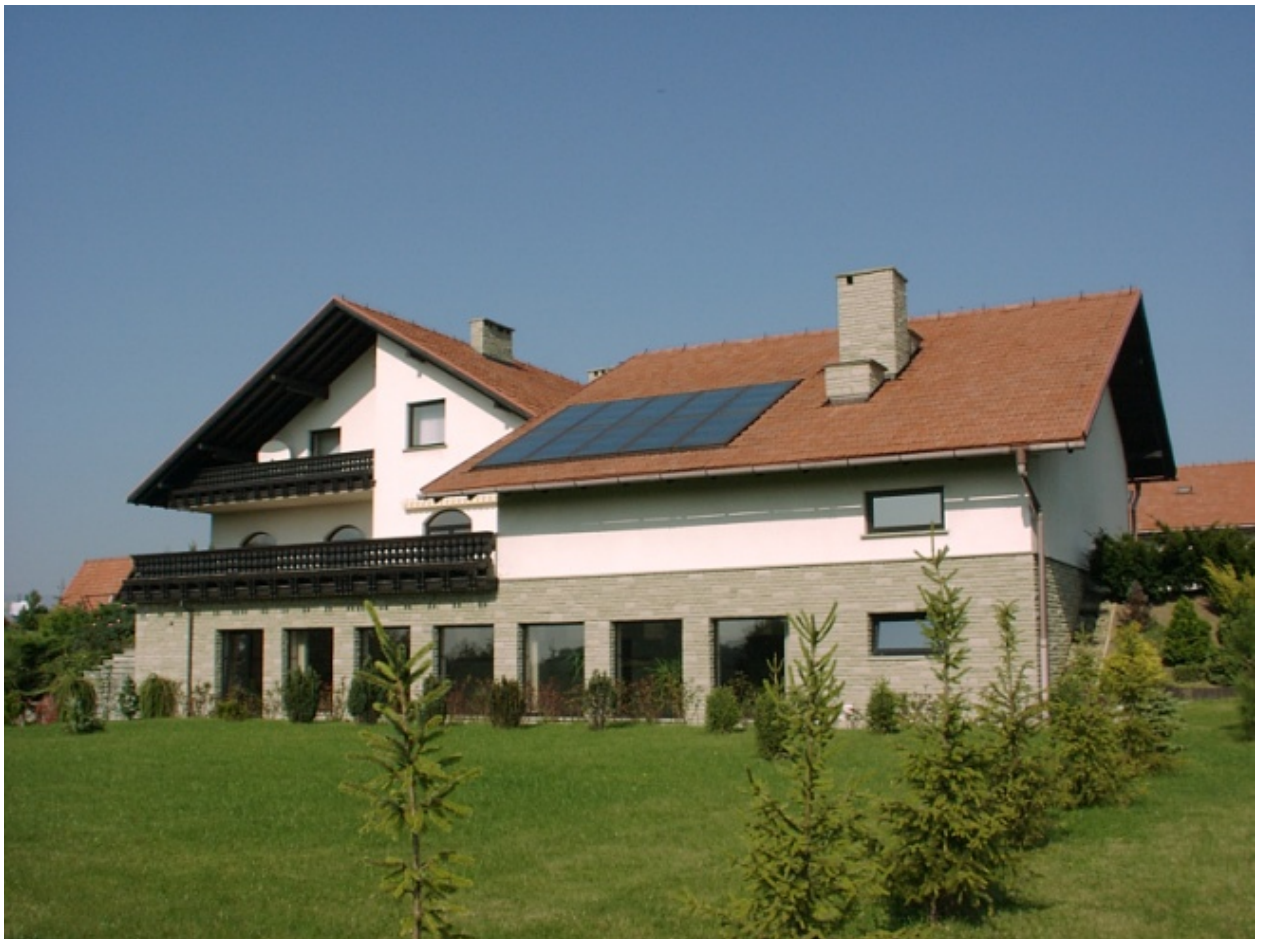
Figure 19 Typical Solar Installation
