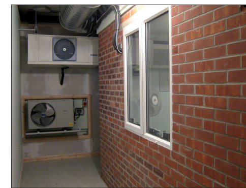
On-site product testing laboratory used internally and externally for product validation and research
