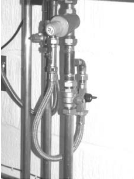
Figure 25: Filling hose connection.
