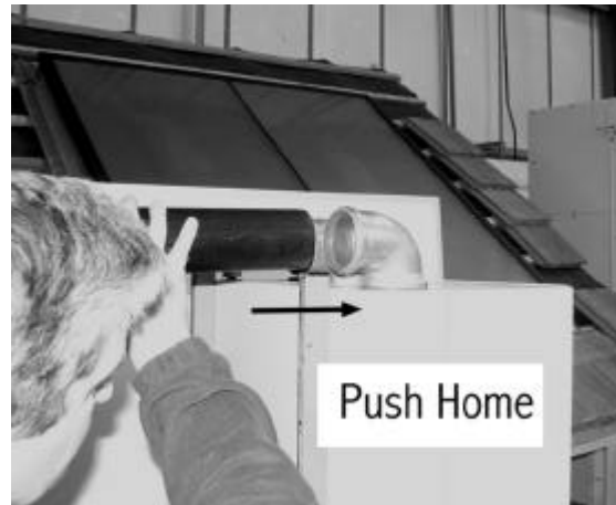
Figure 12: Twin pipe joint
