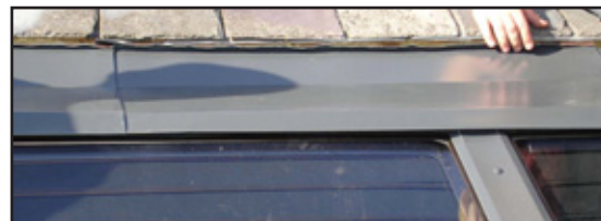
4.6.4.24 (Right) The middle part of the flashing kit side below the left part.
