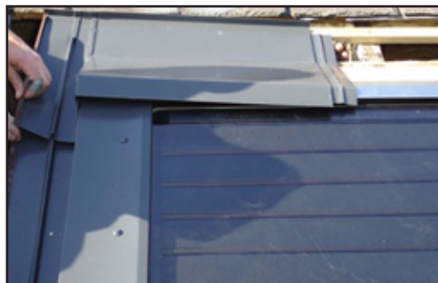
4.6.4.24 (Right) The middle part of the flashing kit side below the left part.
