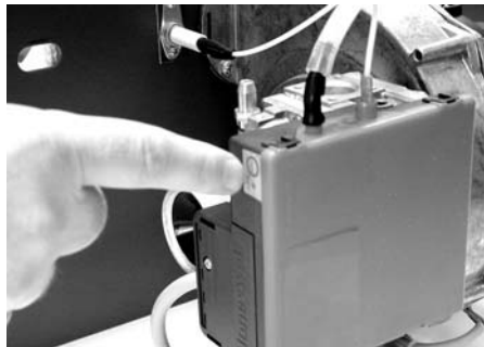
Fig. 25: Gas burner reset button
