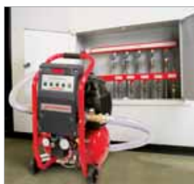
Cleaning of floor heating
