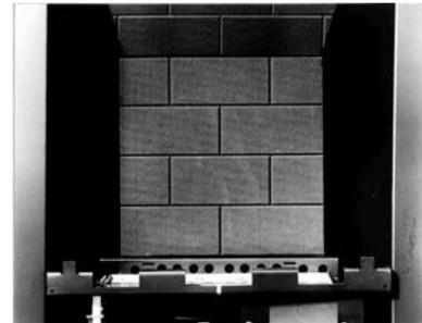
Place the front row of six coals on to the matrix, with the two coals second front each end turned on their sides. Ensure the coals are firmly against the side cheeks as shown in the photograph. If necessary, pull the coals forward slightly to ensure their rear edges do not overhang the flame ports. Corners or rough edges **MUST NOT** be allowed to enter the flame ports. If in any doubt pull the coals as far forward as possible.
