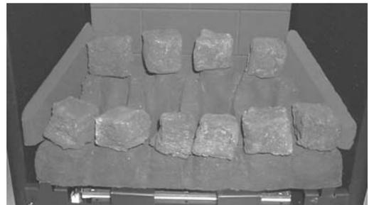
Place the middle row of five coals onto the flats in the matrix. Ensure the coals are not put into the holes in the matrix. Place the two end coals firmly against the side cheeks and back to the steps on the matrix, turning them on to their sides as shown.
