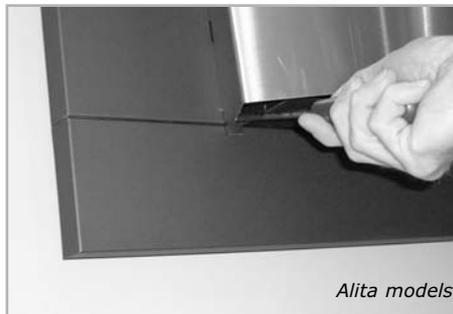
**Alita models** : The front frame assembly simply hooks on to the rear frame at two points. After hooking on the frame, secure it with two fixing screws as shown. The grille is supplied loose and sits inside the top of the frame. Finally, position the shelf onto the support brackets, in front of the glass panel.
