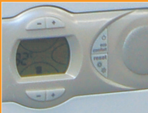
LCD diagnostic boiler fascia panel
