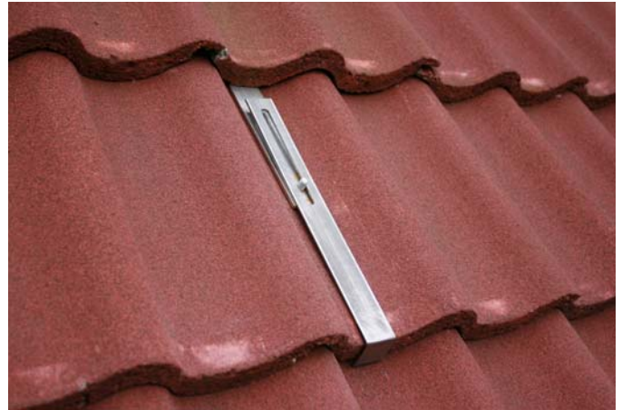
Fig. 12 - Additional support bracket (item 22)
