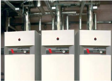
Mutiple unit installations for commercial and industrial applications requiring high volume hot water output
