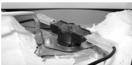
Fig. 26: Safety thermostat reset button.
