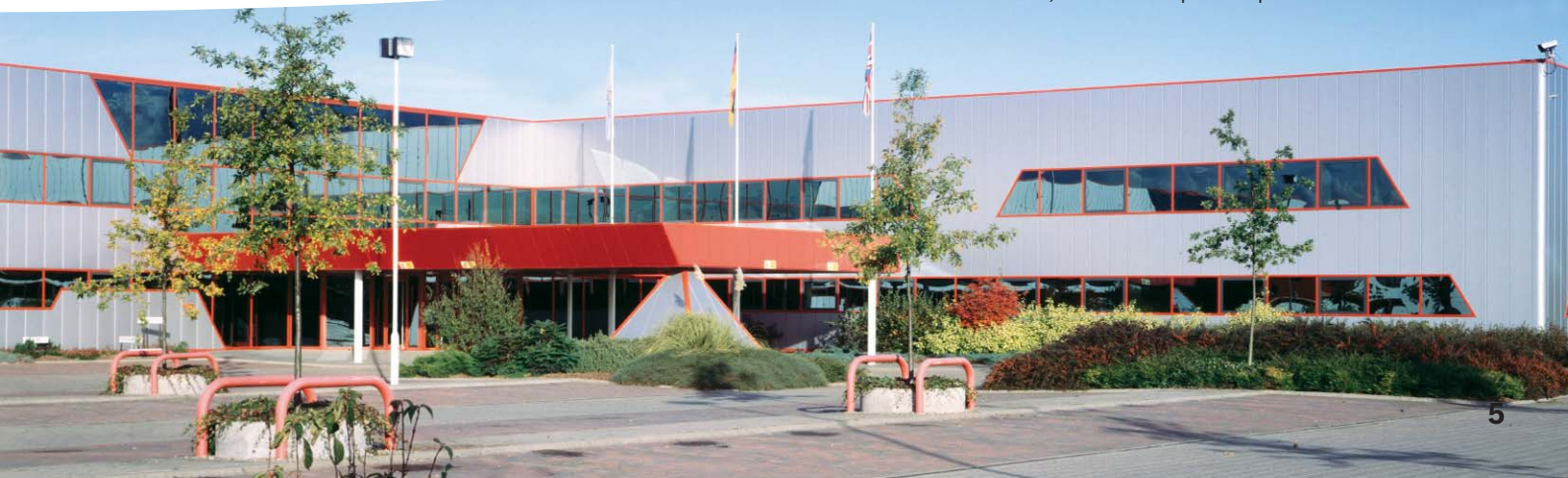
Worcester, Bosch Group headquarters in Worcester
