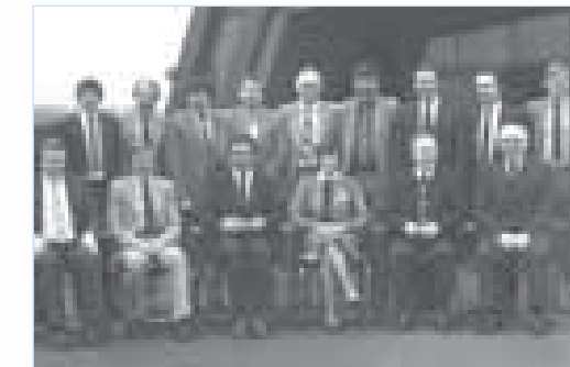
A history of innovation: Worcester introduced the combi boiler to the UK in the 1970s.
