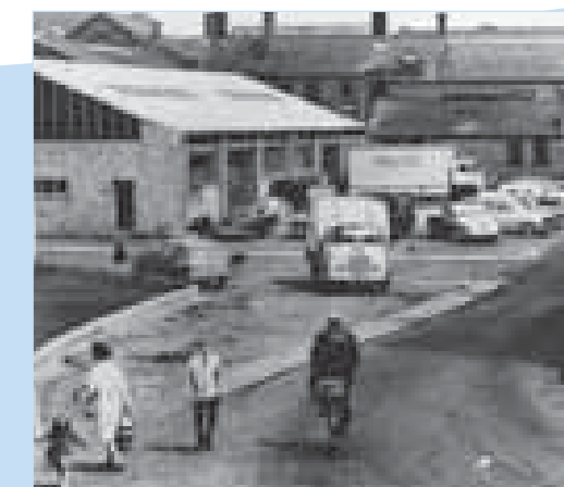
Proud origins: the original Worcester factory.
