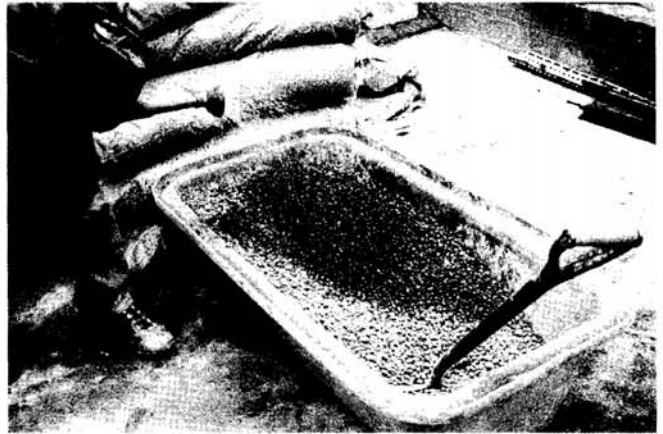
7. Wet the insulation with a small amount of water.
