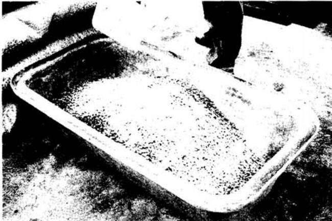
8. Add cement in proportion 1:20 by volume (1 cement : 20 leca) 1 level shovel of Portland cement to one bag of leca..
