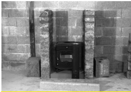
1 Form a chamber in blocks or bricks to suit the stove.
