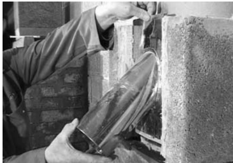
7 Adjust the adaptor pipe to suit the VE pipe from the cooker.
