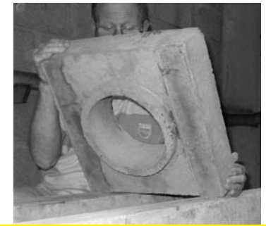
3 Place the support block on a bed of mortar on the heads.
