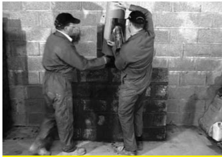
5 Insert the cooker adaptor pipe. Here the 45 degree adaptor is shown but the 90 degree adaptor is also available. The adaptor pipe should be at the same level as the output pipe from the cooker.
