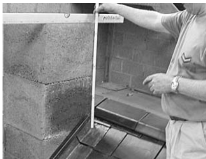
4 Then measure the height of the upper edge.
