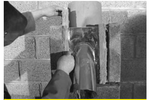
6 Cut and fit insulation around the sides of the adaptor pipe.
