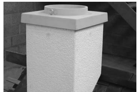
9 Lower the prefabricated stack over the chimney blocks using the sky hooks on the coping. Once in position the sky hooks can be removed.
