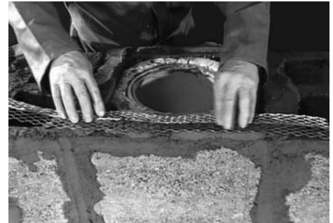
12 Put the supplied expanded metal between the blocks to prevent cracking.
