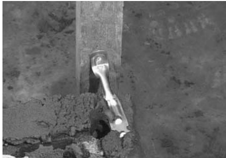
11 Standard timber frame ties should be used in timber frame construction.
