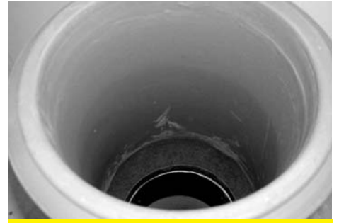
9 Also inside the chimney pot seal the space between the pot and expansion plate with mortar or other non-porous material.
