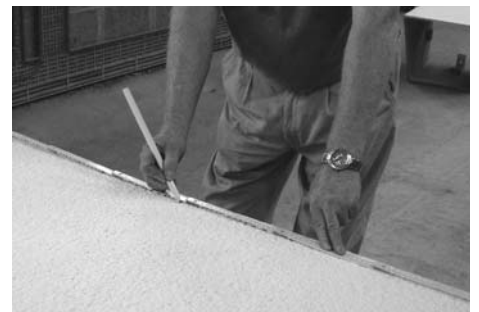
6 And mark out the smaller height on the opposite edge.
