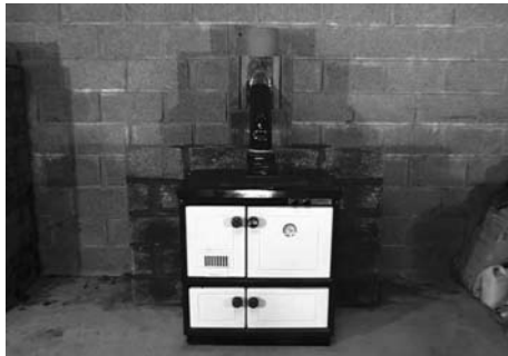
8 Build the chimney system in the normal way.
