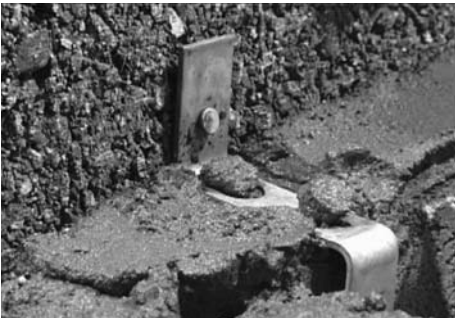
10 The chimney blocks and hollow blocks should be tied every meter to a structural wall with the supplied masonry/steel frame tie.
