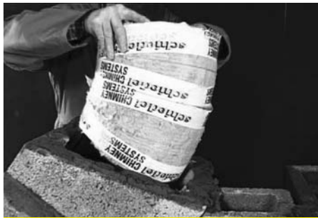
8 Insert the insulated ceramic return bend into the bend block.
