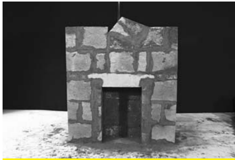
7 Place the straight edge of the third chimney bend block on top.
