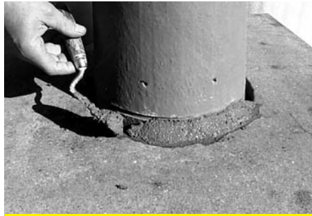
8 Place the chimney pot on the coping ensuring the space between the pot and coping is sealed with mortar or other non-porous material.
