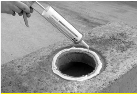
7 Cover the base of the flue aperture in the lintel with high temperature sealant.
