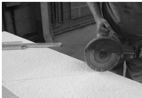
8 Cut the prefabricated stack to the required height. The stack shown here is for a roof slope. A similar procedure should be followed for a stack at the ridge.
