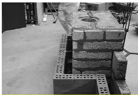
5 Seal between the lintels with mortar.
