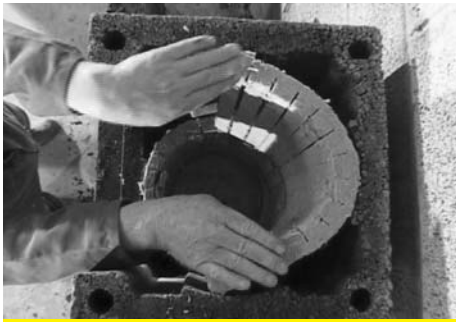
4 Insert the insulation.
