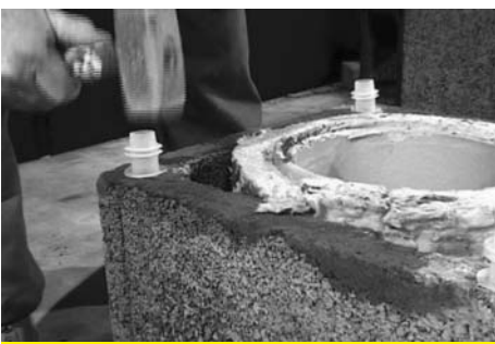
16 Continue to build the chimney as a single block to the stack. Special plastic connectors are inserted in all 4 corners of the chimney block to provide stability against wind loading. These should be used from a point 1 meter below the last point of lateral support.
