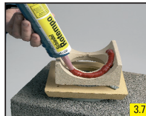
3.7 Apply Schiedel High Temperature sealant onto inner connection piece.
