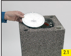
2.1 Place the joint protection cover onto the profiled pipe to stop mortar falling into the pipe.
