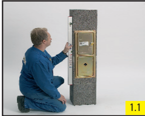
1.1 Prepare mortar bed, set prefabricated base in mortar.
