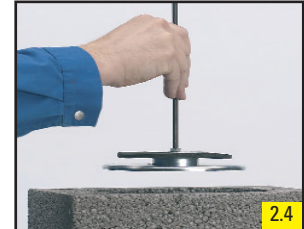
2.4 Remove joint protection lid with magnet on the joint smoothing tool.
