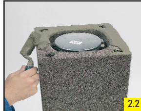
2.2 Apply thin-bed mortar.
