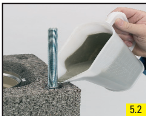
5.2 Pour the mortar into the reinforcement ducts. Pay attention to even axis distances.
