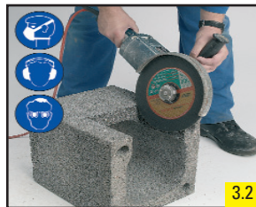
3.2 Cut opening for connection piece with angle grinder.
