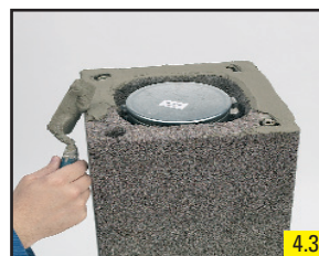
4.3 Apply thin-bed mortar.
