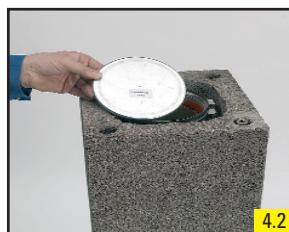
4.2 Put joint protection cover onto the profiled pipe.
