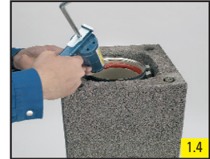
1.4 Apply Schiedel High Temperature sealant generously in the sleeve of the profiled pipe.
