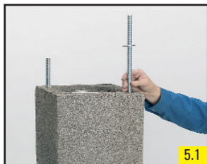
5.1 Insert stoppers on underside of block. Screw two reinforcement rods together and insert them diagonally.
