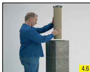
4.6 Insert profiled pipe (L = 66 cm).
