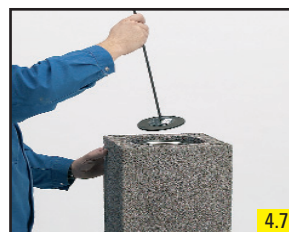
4.7 Float profiled pipe joint with joint smoothing tool.
