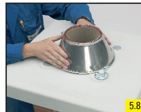
5.8 Slide cone over the pipe until it sits on the cover plate.
