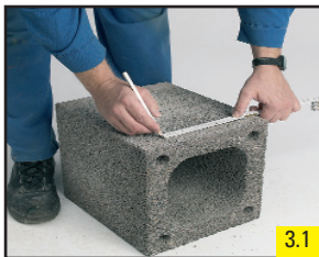
3.1 On the outer block opening mark 21 x 21 cm.
