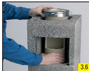
3.6 Insert profiled pipe.
