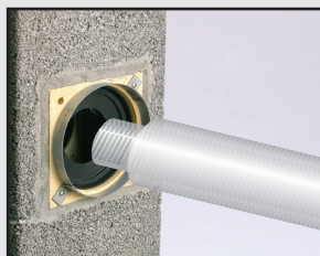
Smear the connection pipe with a lubricant and then slide the pipe into the adapter.
