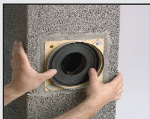
Insert plug-in adapter(s).
