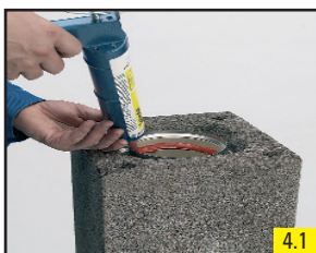
4.1 Apply Schiedel High Temperature sealant generously onto the profiled pipe.
