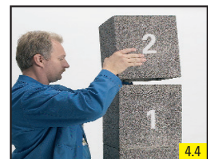
4.4 Set two outer blocks. The blocks should be tied every metre to a structural wall.
