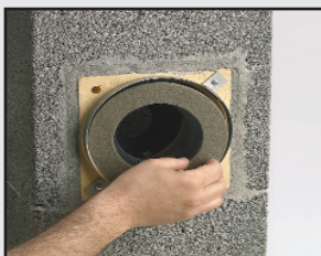
Insert insulation ring.
