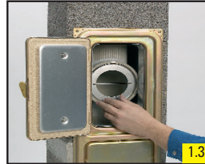
1.3 Insert overflow brake from the MULTI package.
