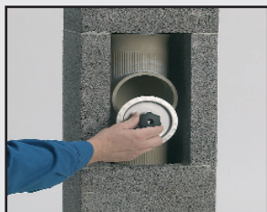
Insert inspection cover.
